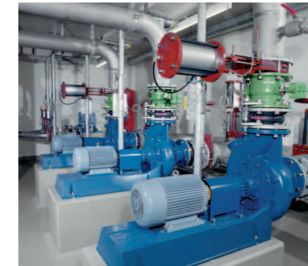
Pumps installed horizontally on a baseplate for fast service.
